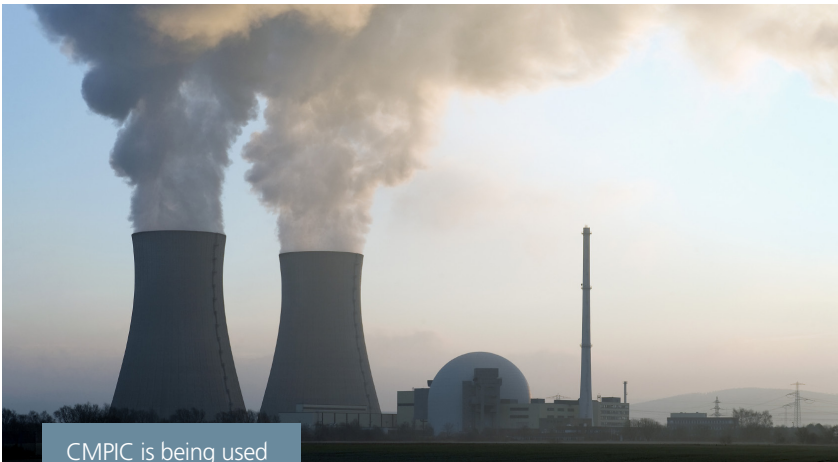
CMPIC is being used in the design of nuclear and thermal power stations
